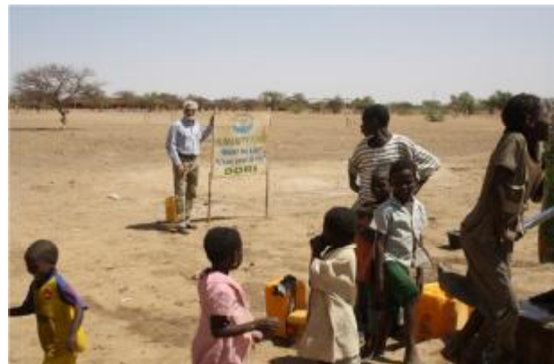
Hand pump for water in Dori, Burkina Faso installed by Humanity First under "Water for life" program.
